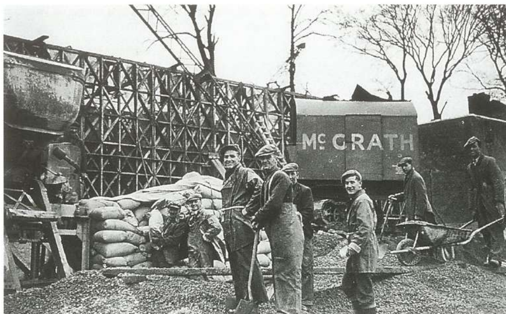
McGrath workmen on-site.
